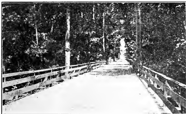
BRIDGE (900 FT.) ACROSS LAKE CHUMUCKLA.
